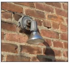
3. The light fixtures serving the laundry room are controlled by manual switches. Therefore, these lights are often left on when this space is unoccupied.
