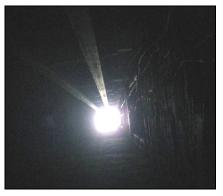
The attic has been insulated but not air-sealed. Numerous air leakage points exist, particularly between the brick structure and wall framing at the exterior perimeter and around the stairwells. Additional leakage points exist at the tops of partition walls and around the chimney and dumbwaiter chases.
