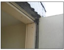
Caps are fitted to the peaks of the skylights that illuminate the top of the stairwells. These caps appear to be open at all times, possibly to provide corridor ventilation. However, they are a significant source of winter heat loss.
