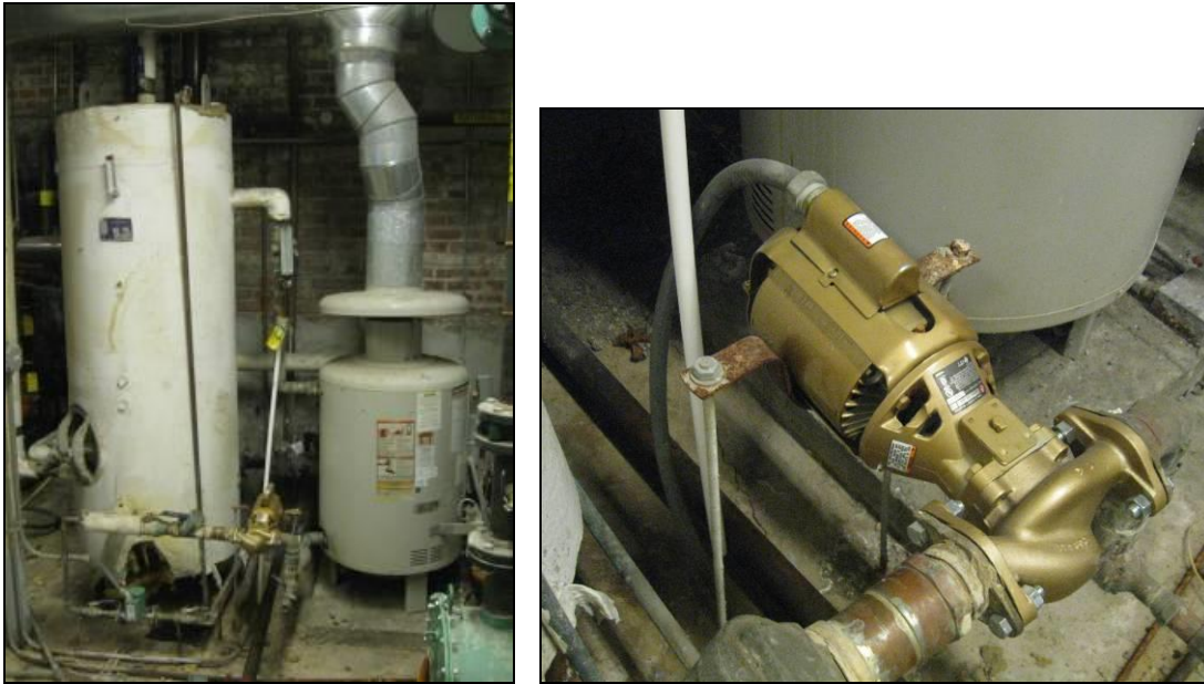
Domestic Hot Water System and Boiler Circulator Pump
