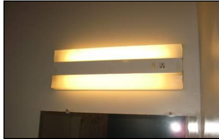
Apartment Bath Light Fixture
