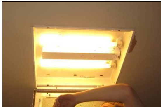
Corridor Light Fixtures
